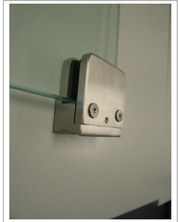
Loosen enough so the Screw Heads project above the Clamp
